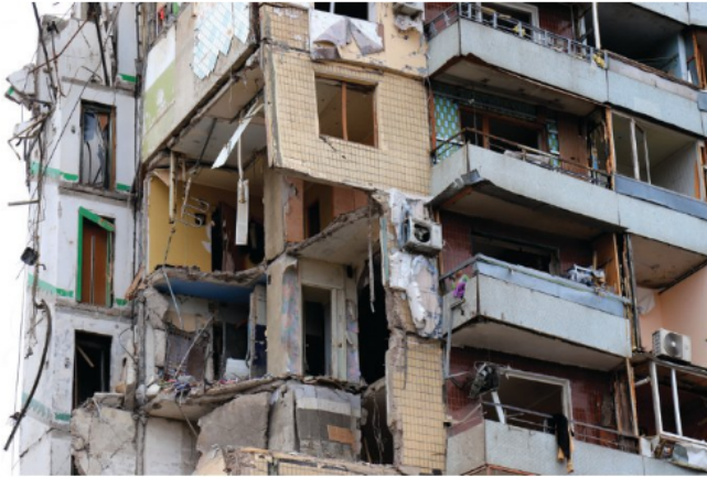
■ Figure 4.24 The impact of war on civilians: this apartment building in Ukraine was destroyed by a Russian missile strike
